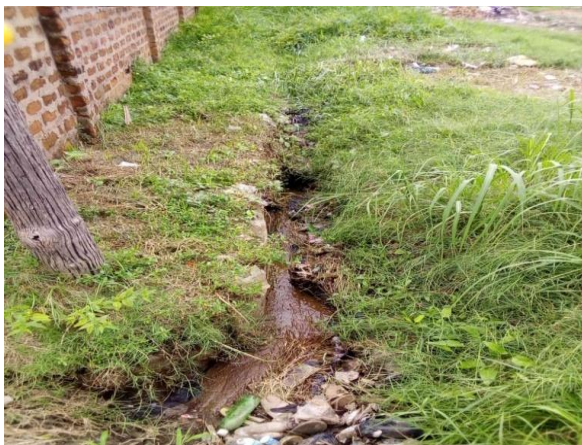
Figure 5: A drainage channel covered with vegetation
